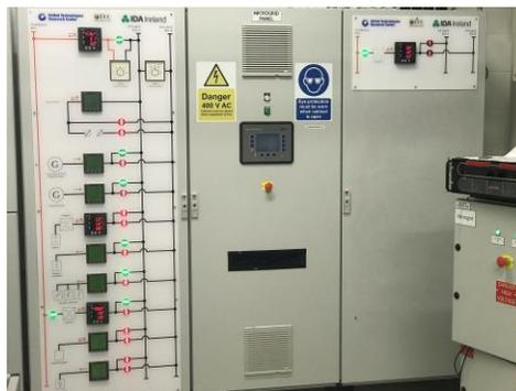
Figure 3: MaREI microgrid distribution panel
